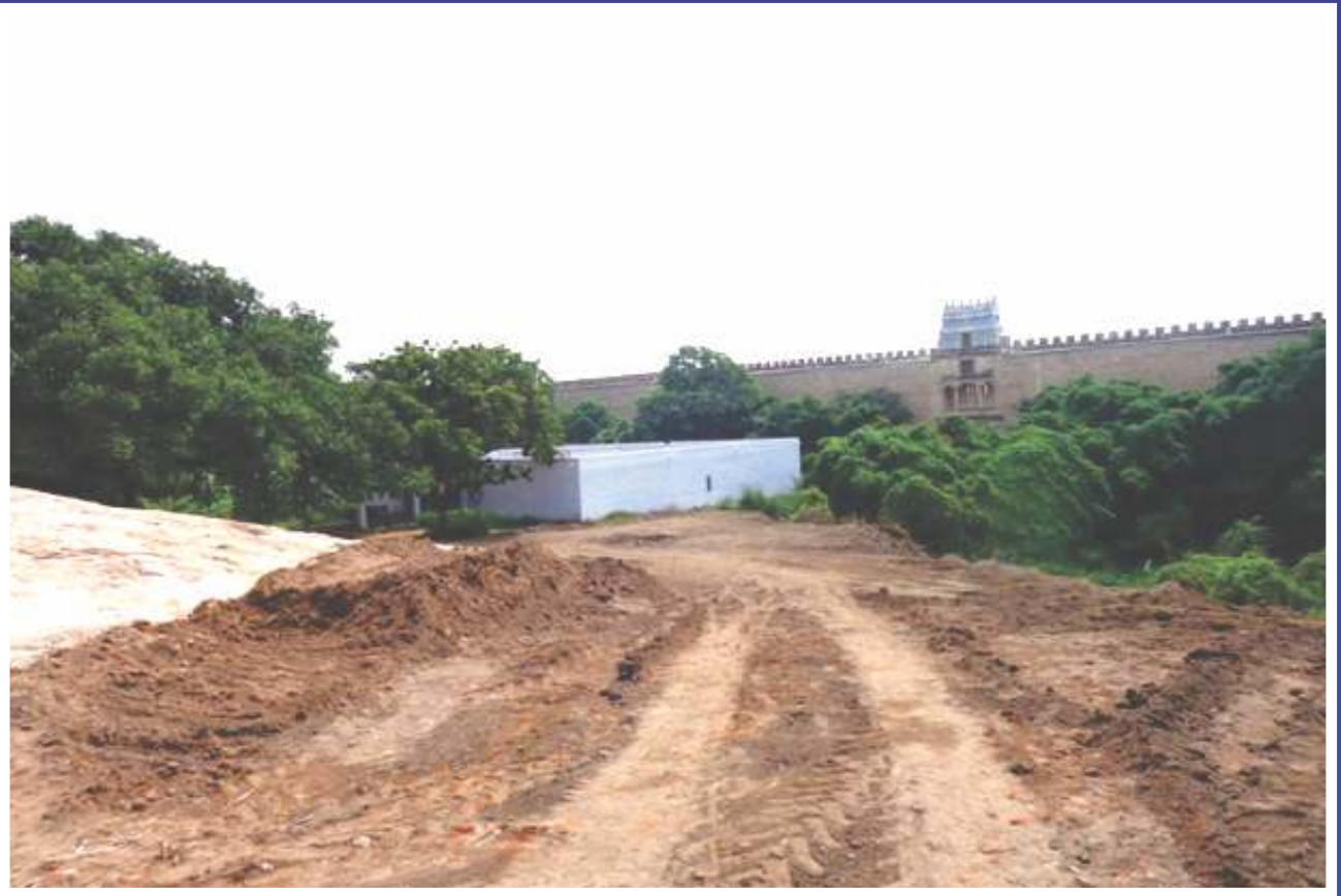
South west prakaram - Before renovation
