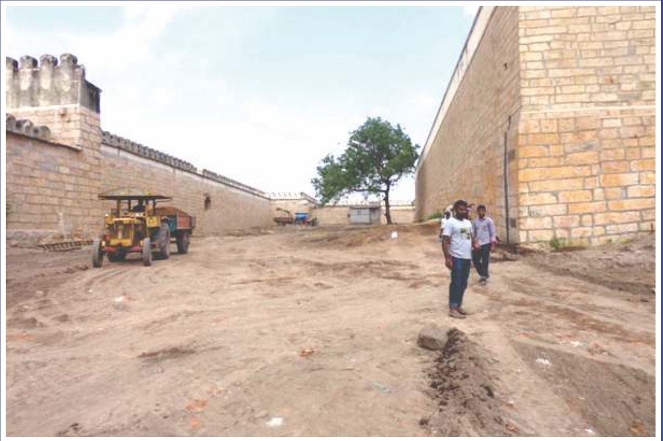
West prakaram - Before renovation
