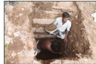
Figure 5: Trial pit at location 2 in progress
