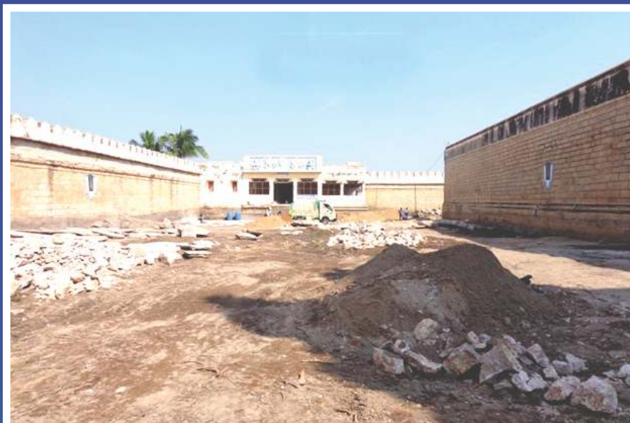
North prakaram - During renovation
