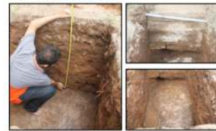
Figure 6: Trial pit at location 1
