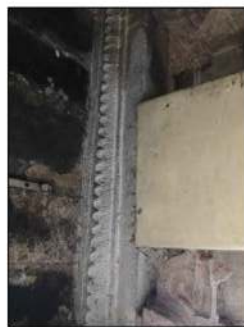
Figure 4: Deteriorated timber members
