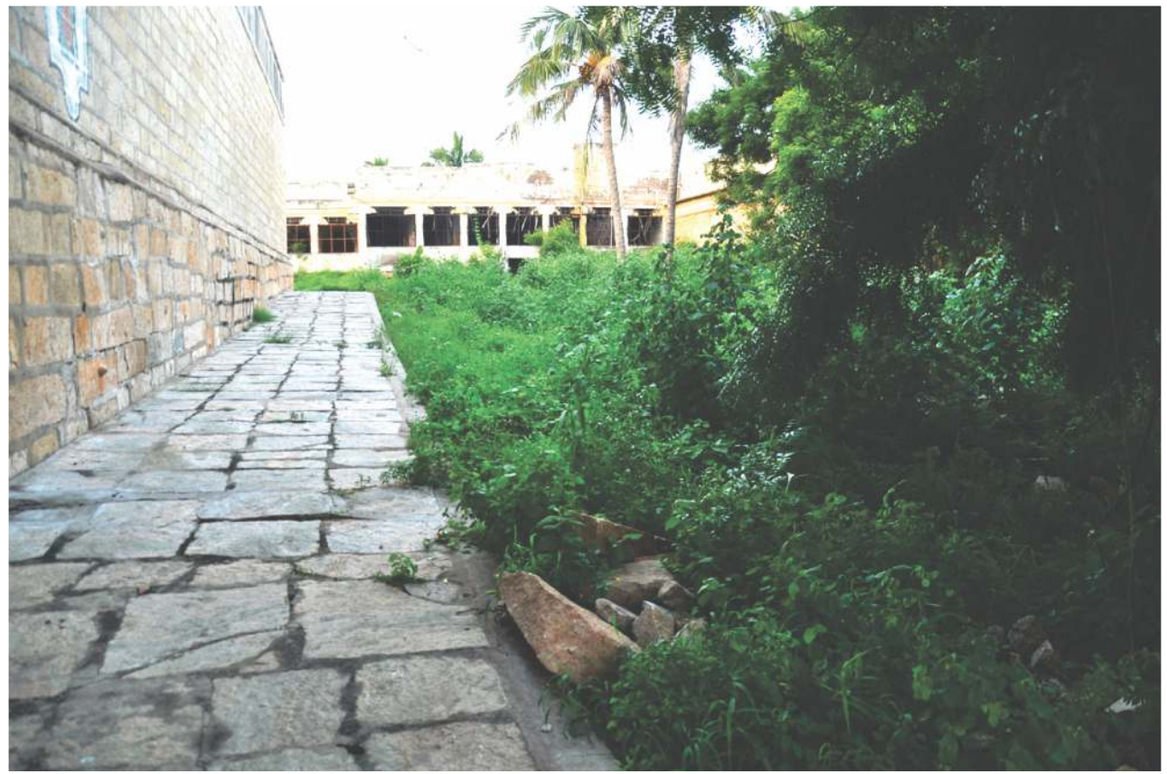
East prakaram - Before renovation
