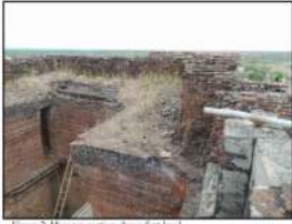
Figure 2: Masonry section above first level
