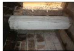
Figure 12: Masonry pier as temporary support
