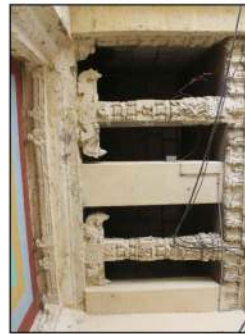
Figure 14: Masonry pier as temporary support at upper level
