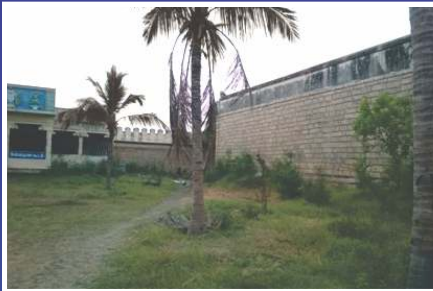
North prakaram - Before renovation
