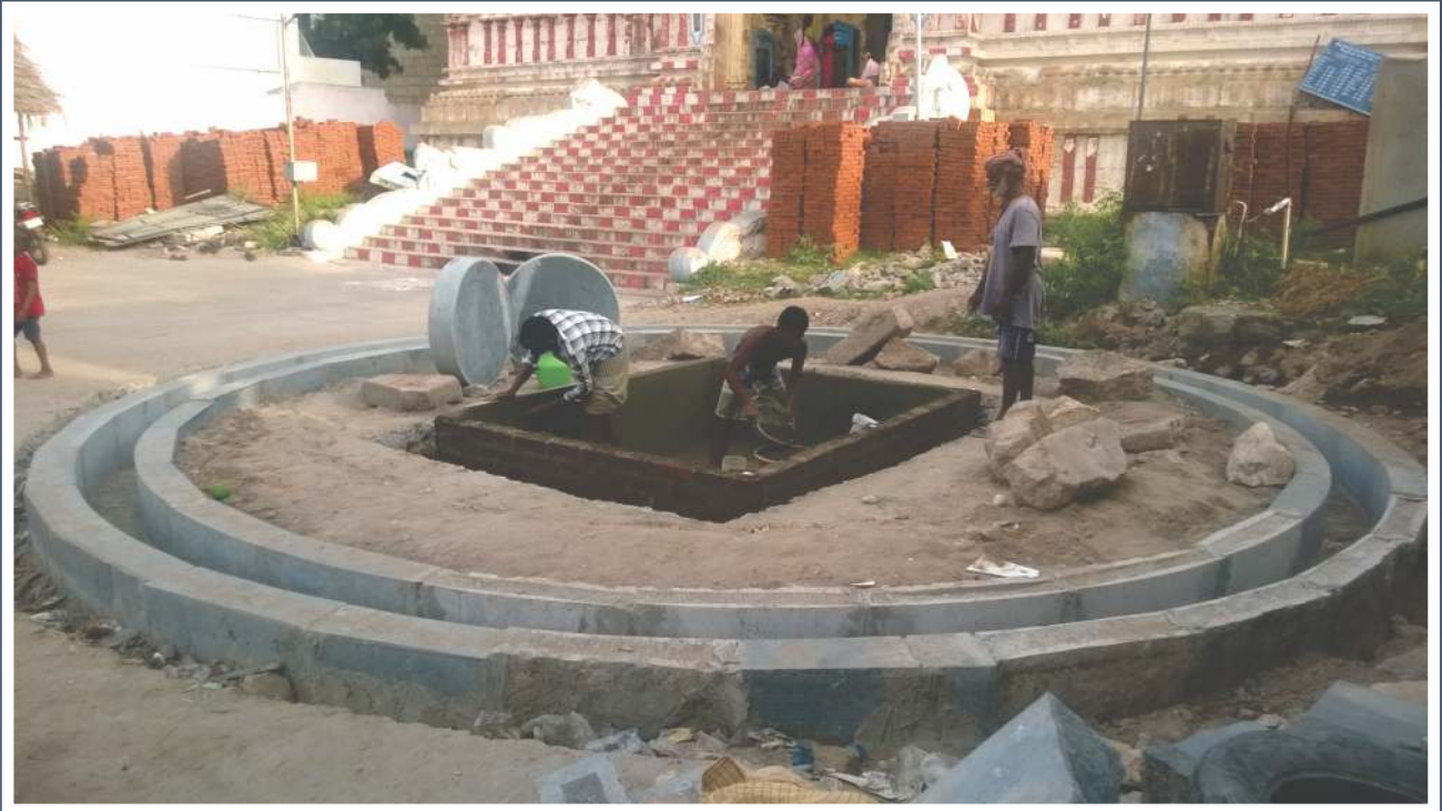
Traditional lime mortar preparing arrangement in process
