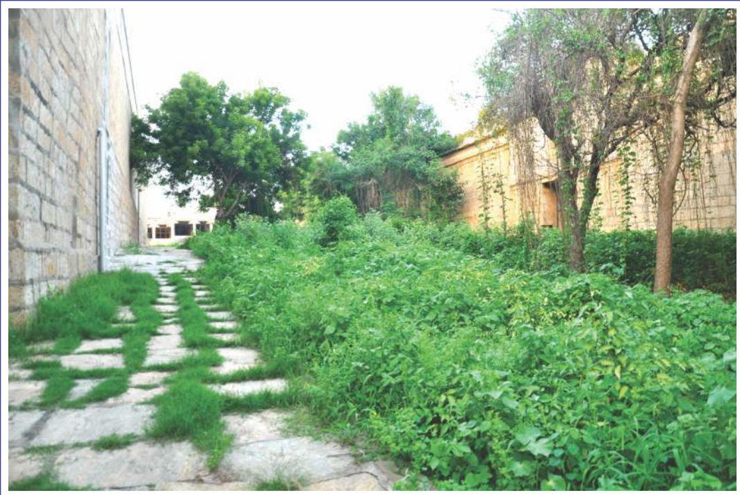
East prakaram - Before renovation
