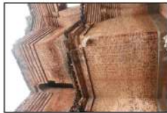
Figure 4: Deteriorated timber members
