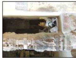
Figure 6: Deteriorated and abandoned masonry in upper floor.
