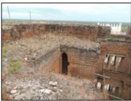
Figure 3: Masonry section above first level
