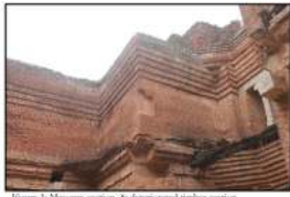
Figure 1: Masonry section & disintegrated timber section
