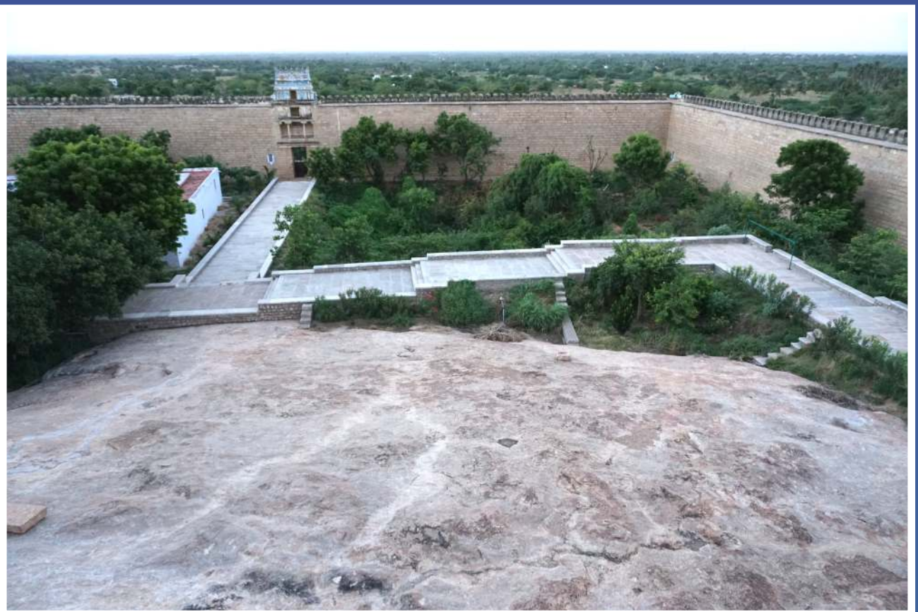
South west prakaram - After renovation
