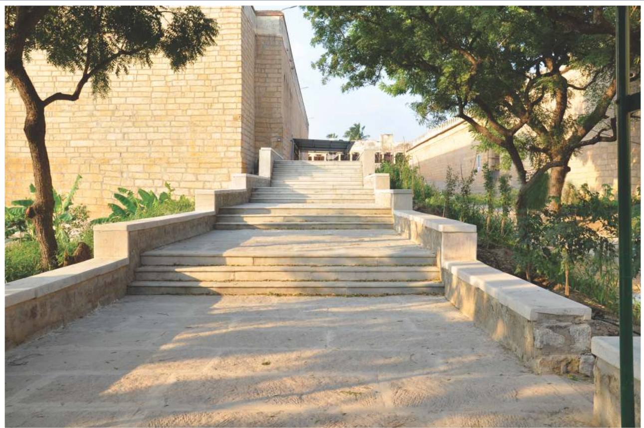
East prakaram - After renovation
